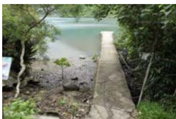
The pier near the chapel
