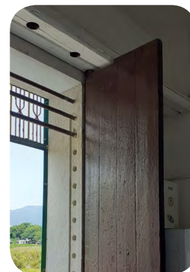
Holes remained of the original shutter
