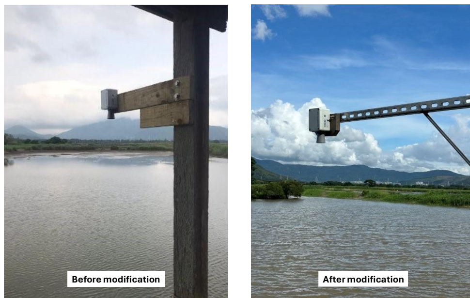
Figure 10. Water level sensor and its supporting infrastructure before and after replacing supporting materials
