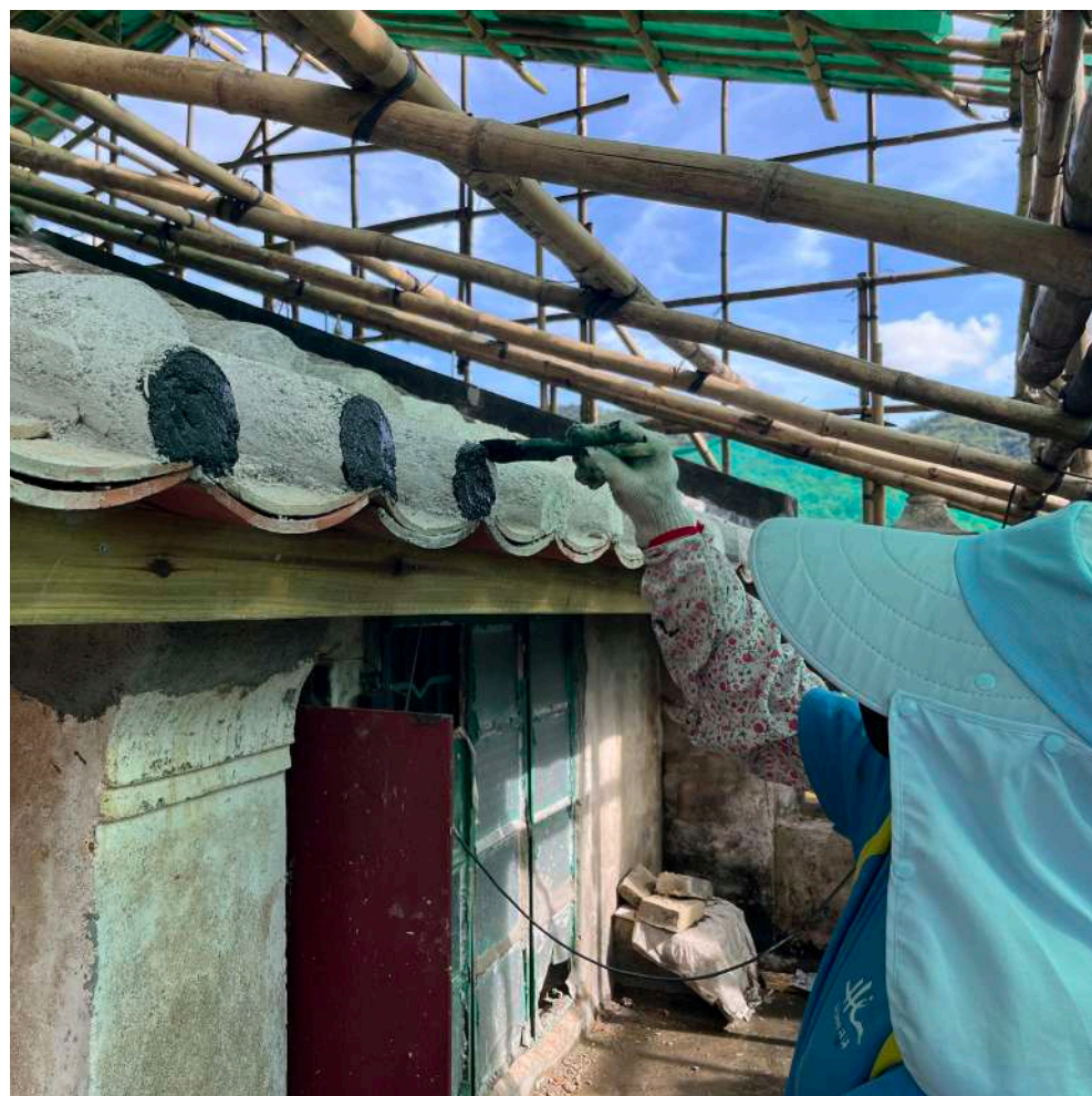
重做瓦頭和上油 Remake Lime end-stopper
