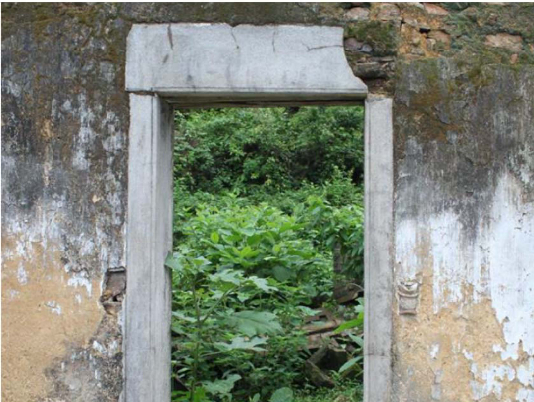
Rammed earth + Granite + earth plaster + cement screeding
