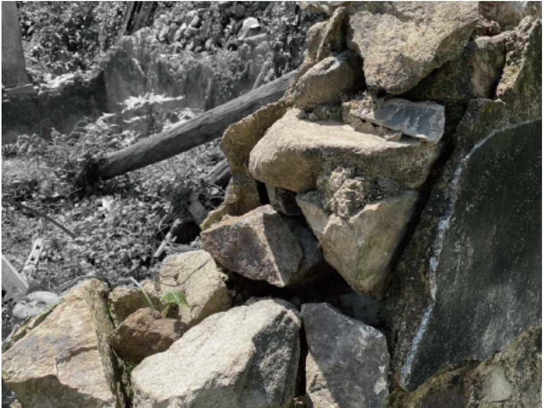
Earth mortar + Plaster
