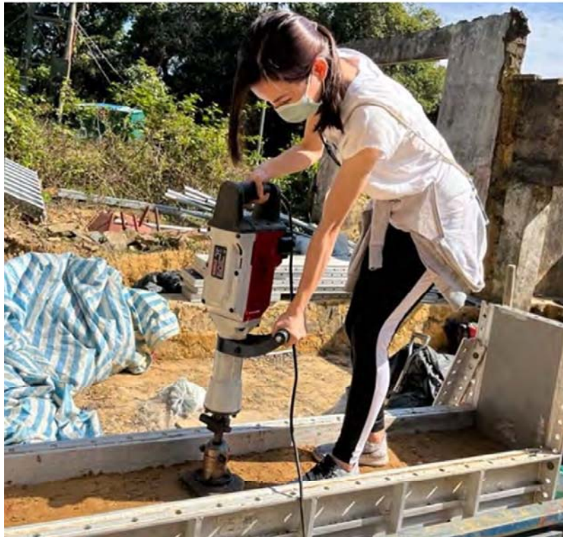
Construction of rammed earth wall in 2022
