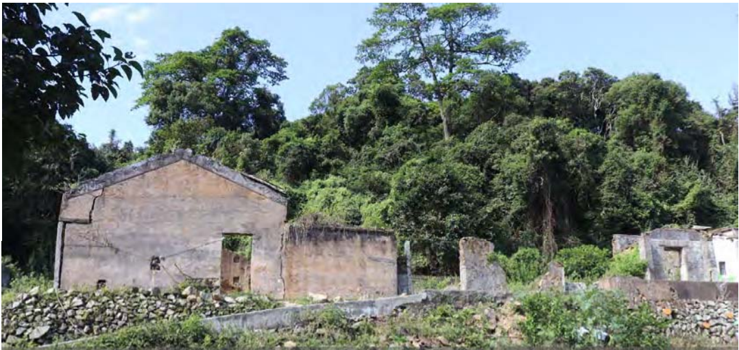
Rammed earth wall of the Old House
