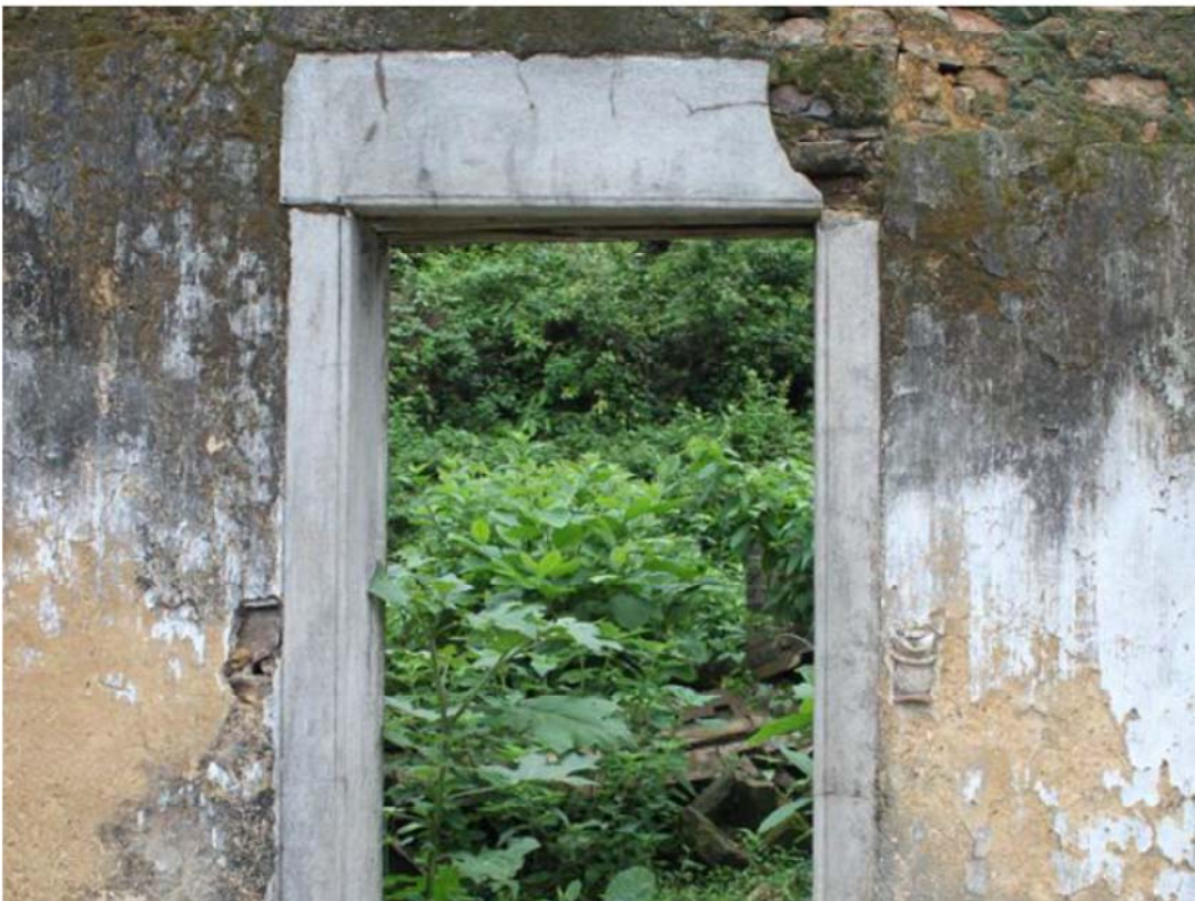
Rammed earth + Granite + earth plaster + cement screeding
