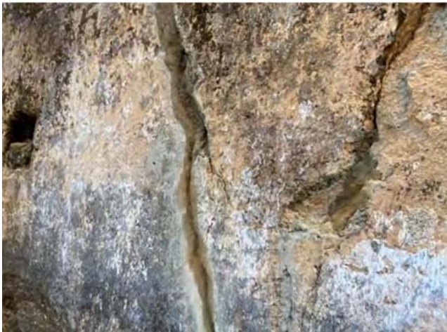
Filling up the crack with cement, sand, soil and nails
