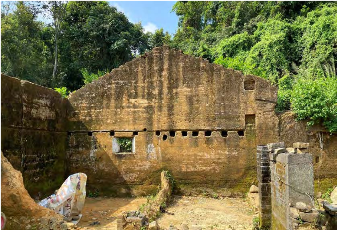
Rammed earth wall of the old house
