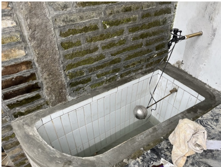
Ball valve installed to control water flow into the restored water tank
