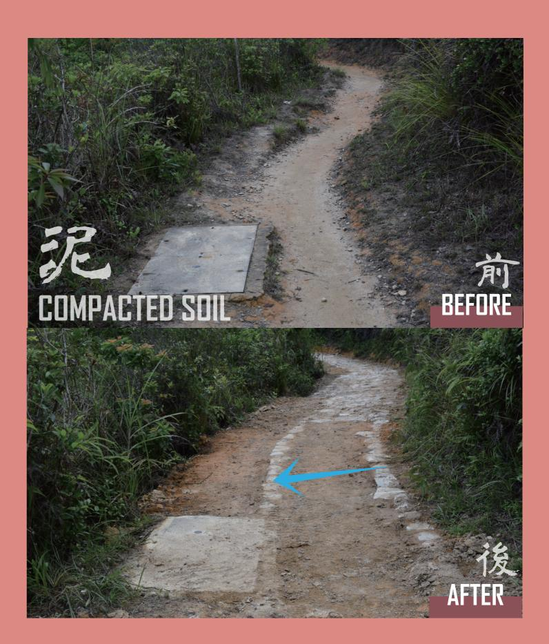
試驗性修復大埔郊遊徑 EXPERIMENTAL INSTALLATION OF STONE SLABS in TAI PO COUNTRY TRAIL
