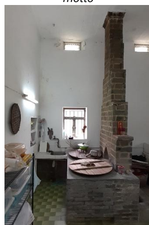
Fig. 4.11- Brick stoves and chimney
