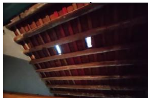
Interior side during the water test- no seepage is found
