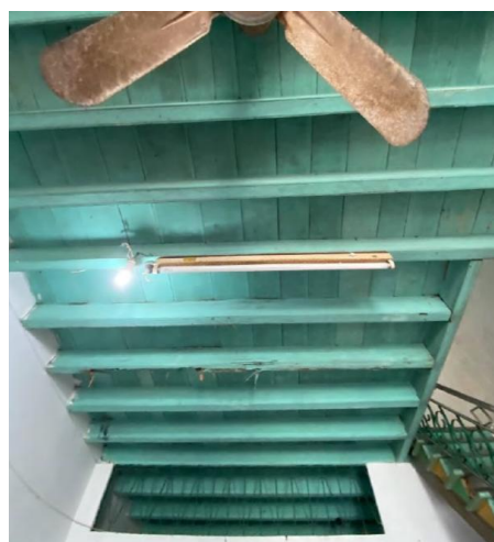
Fig. 2.16- Before restoring the joists of cockloft
