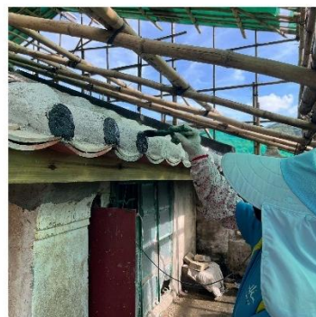
重做瓦頭和上油 Remake Lime end-stopper
