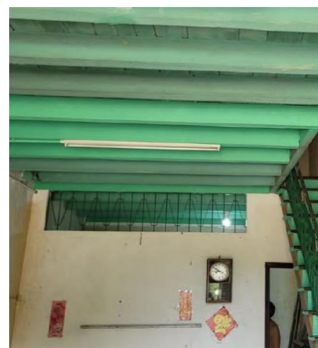
Fig. 2.17- Restoration of cockloft joists with Kapur
