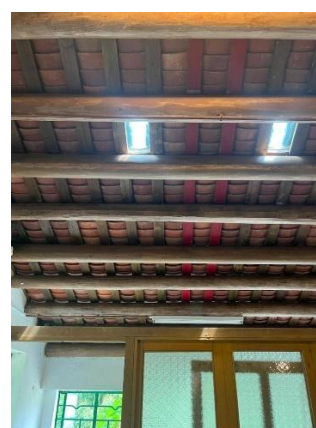
Fig. 2.7- Timber battens and purlins with skylight roofing
