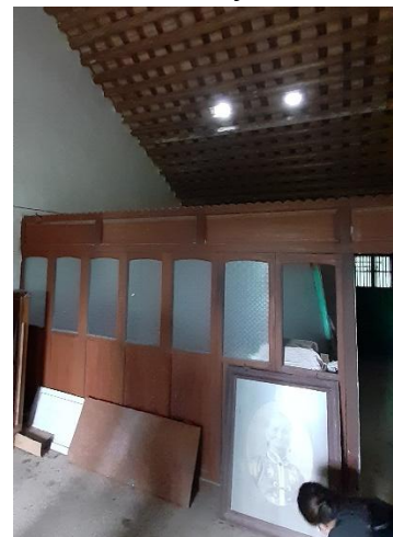
Fig. 5.5.8- Timber partitions on 1/F
