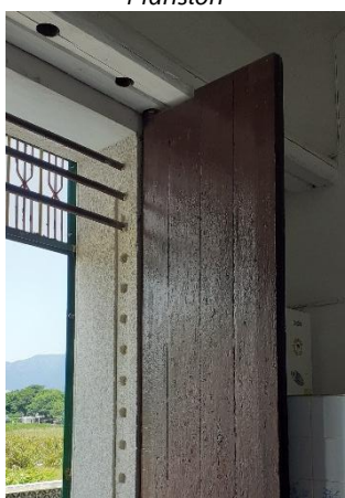
Fig. 4.10- Holes remained of the original shutter
