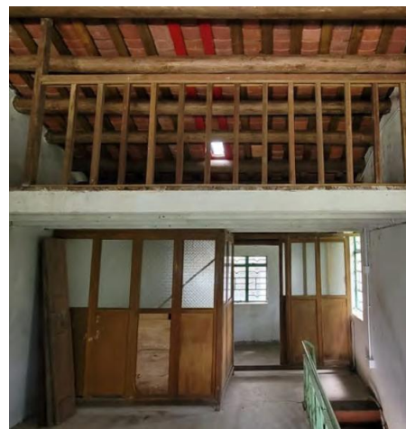
Fig. 2.15- Restoration of roof purlins with Chinese fir
