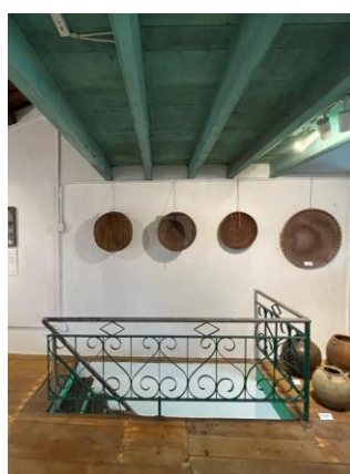
Fig. 2.6- Timber planking of cockloft and staircase rail
