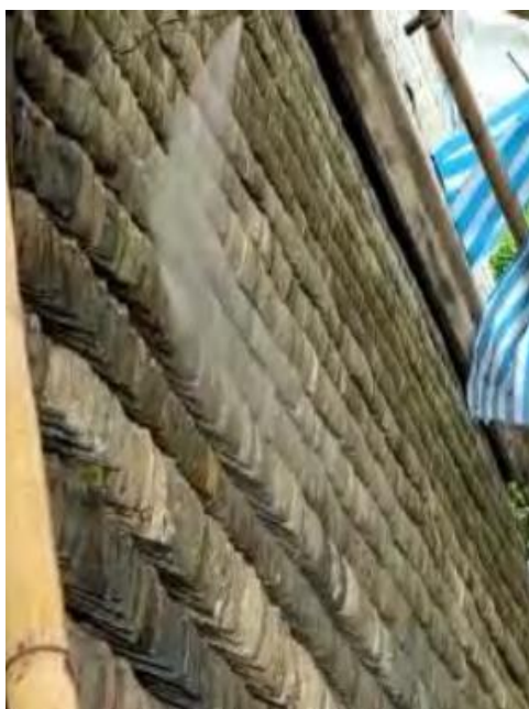
Spraying water onto roof surface at front bay
