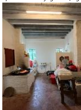
Fig. 2.10- Plastered brick stoves in the right bay
