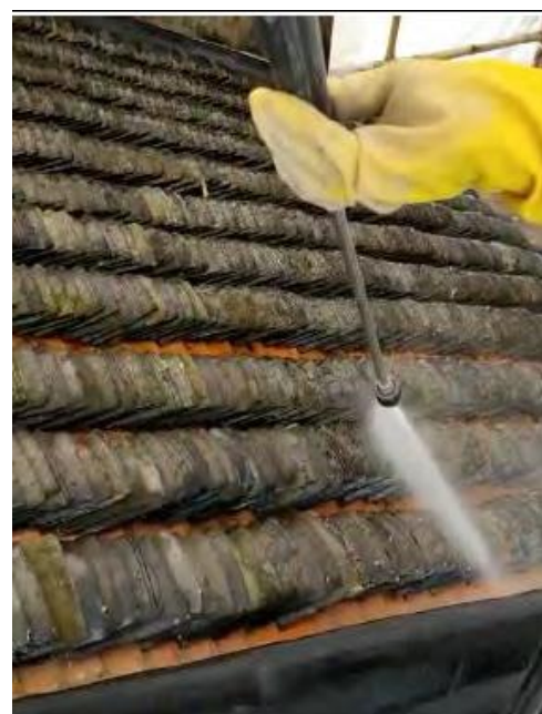
Spraying water onto roof surface at back bay
